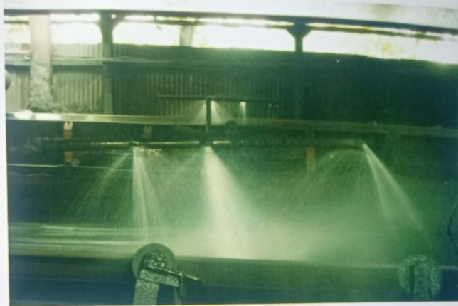
BELT CONVEYOR OF CHP
